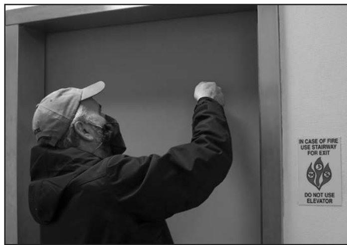
Josh Blatchley, facilities director at the school district, uses a tool to open the door to the high school elevator, which has been out of operation since March of 2020 due to an oil leak. The borough plans to replace the elevator.
