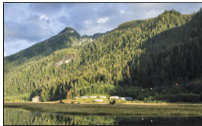
Tyee Lake Hydroelectric Project
